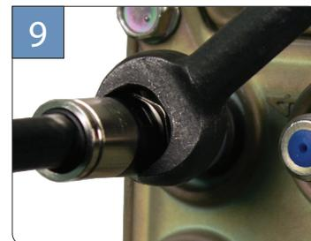
Tighten connector to recommended torque.
