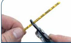
2. Using strippers remove approximately 50mm / 2" of cable jacket.
