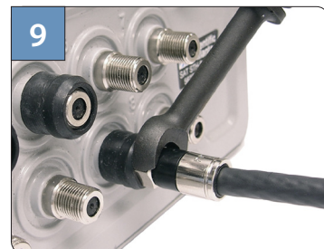
Tighten connector to recommended torque.
