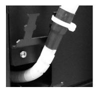
6. Secure feeder cable to cable entry clamp using supplied hose clamps or other suitable fastener like a zip-tie.
