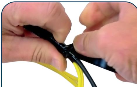
2. Secure mesh edge with tape, catching a small amount of the cable (approximately 1 inch).
